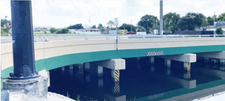
NW 34th Avenue Bridge Improvement
