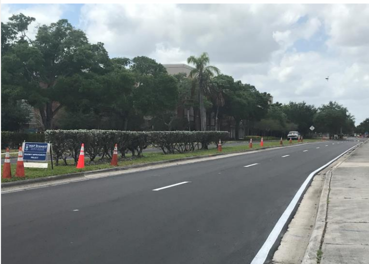
Plantation Roadway Resurfacing
