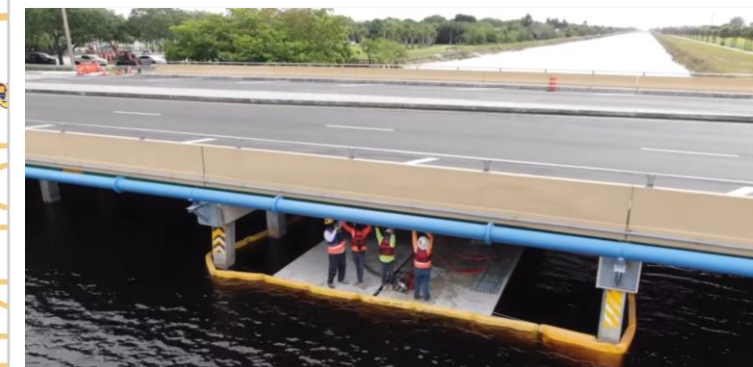
Flamingo Road Bridge Improvement
