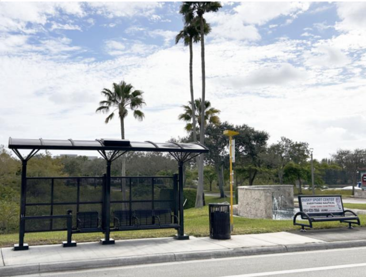
Anglers Ave & Gulfstream Way Bus Shelter
