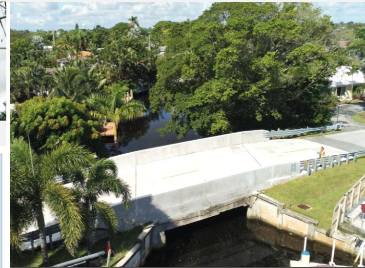
SE 13 th Avenue Bridge Maintenance
