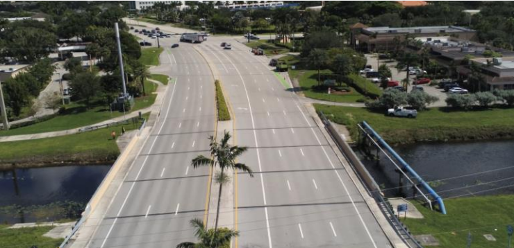
Oakland Park Boulevard Bridge Improvement
