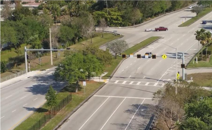
Flamingo Road Intersection Improvement
