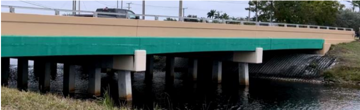
Flamingo Road Bridge Improvement
