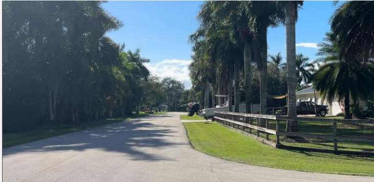
Southwest Ranches Road Rehabilitation and Resurfacing
