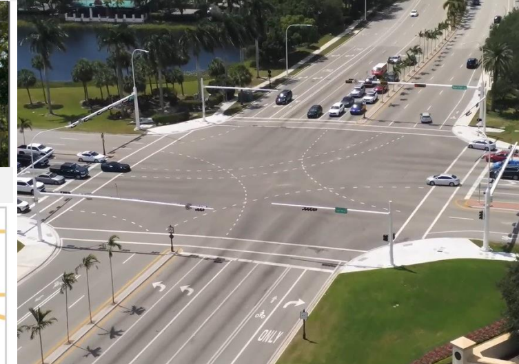
Royal Palm Blvd and Weston Road Intersection Improvements
