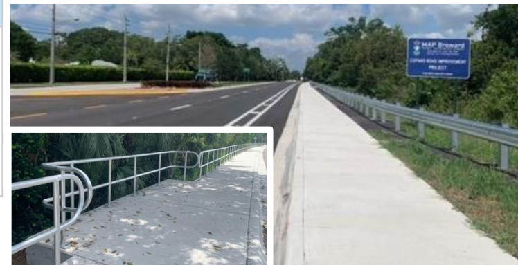
Copans Road Sidewalk Improvement
