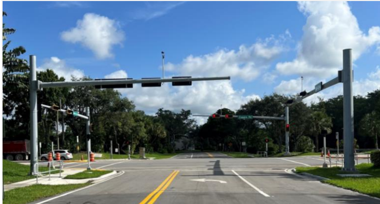
Copans Road and NW 42 nd Mast Arm
