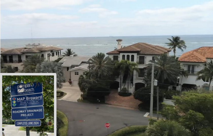
Bay Drive Drainage Improvement
