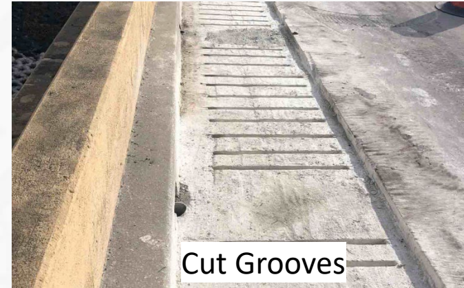
Mark Location of New Steel Rebars
